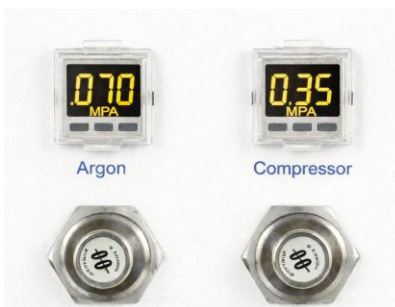
Figure 5-1: Verify compressor pressure readings
